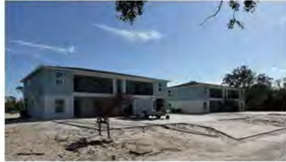
Construction continues on three multi-family quadruplexes located on Fox Hollow Drive.
