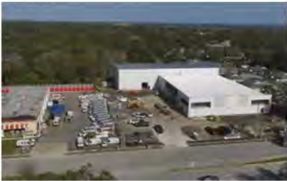
Construction continues on a 16,157-square-foot warehouse and 44,238-square-foot self-storage building at 2060 Garden St.
